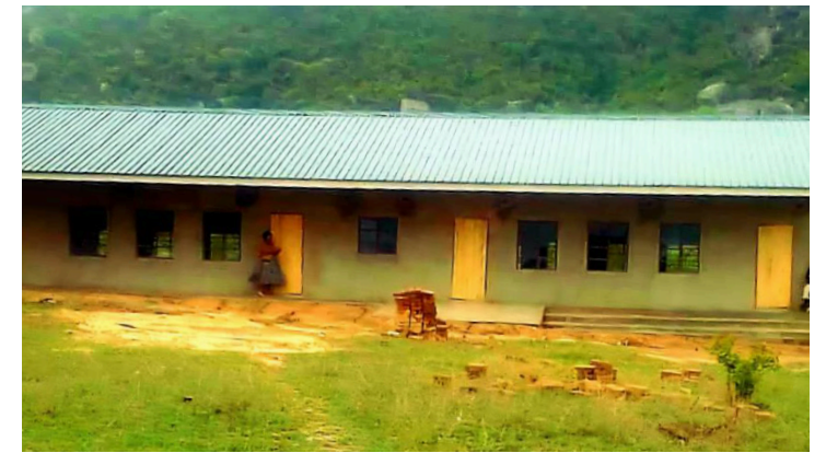
Completed building with roof, plastered walls, doors, and windows in place
