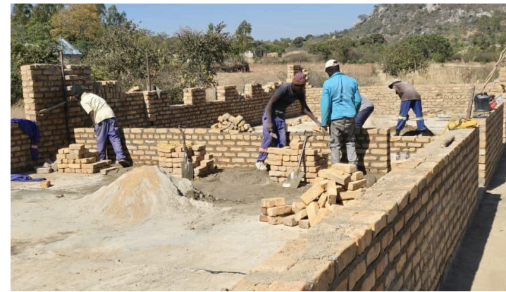
A team of masons laying brick walls together on the foundation slab of St. Bernard's School
