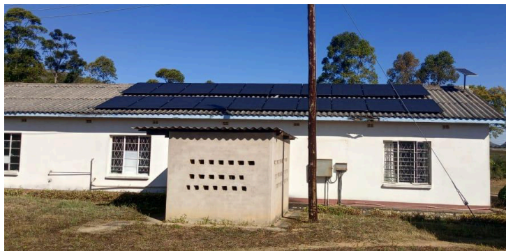
St Barbara's Mission Hospital with solar panels installed on the roof.
