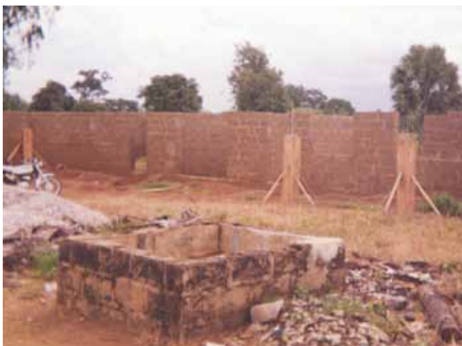
Foundation Walls Recently Erected for the New Classroom Extension in Kaduna
