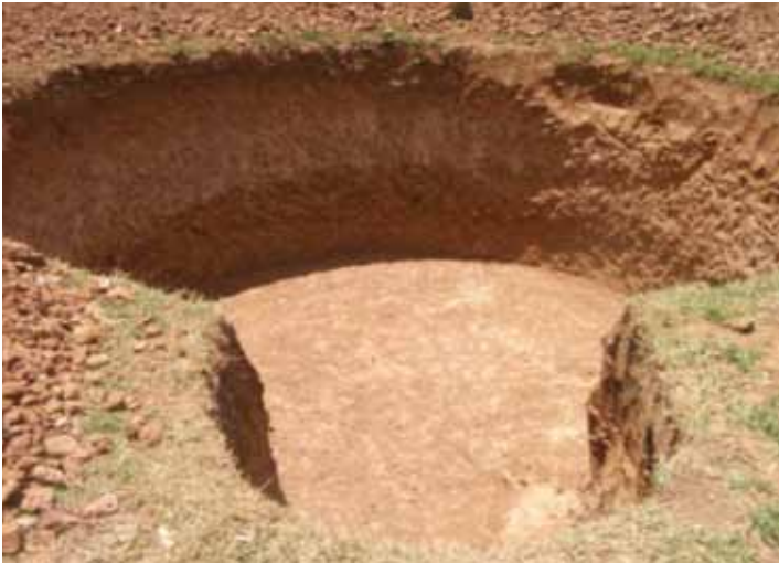
The large hole is now ready for the cement and brick foundation.
