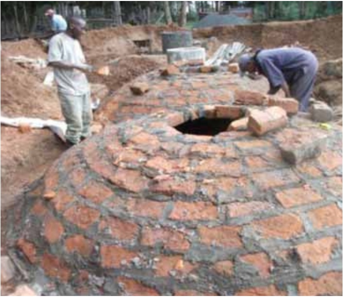
The caps are being cemented in place.
