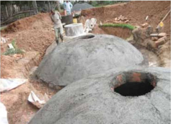
After a final layer of cement is placed over the caps, circular cement moulds are fitted.
