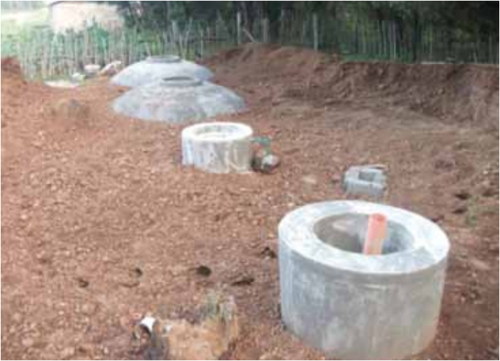
With the moulds in place, the digester beds are recovered with dirt. Pipes to carry the biogas to the nearby buildings are now in place.
