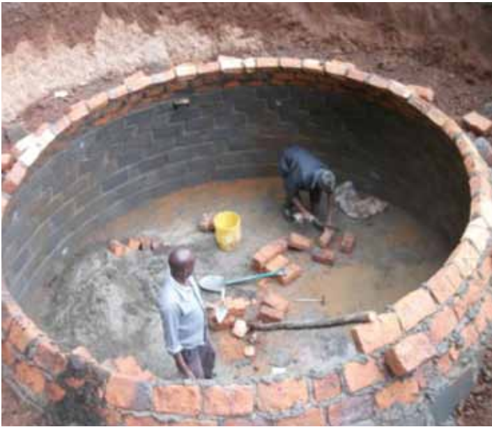
Thick bricks, tightly sealed are built in an igloo shape inside the cavity. It is essential that the digester be properly sealed to prevent leakage and possible contamination of the local water table.
